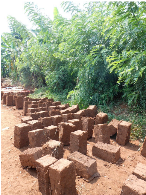
Figure 18: Bricks made by the association for one member to build houses on the family plot (photo by Jennifer Ilo Van Nuil)
